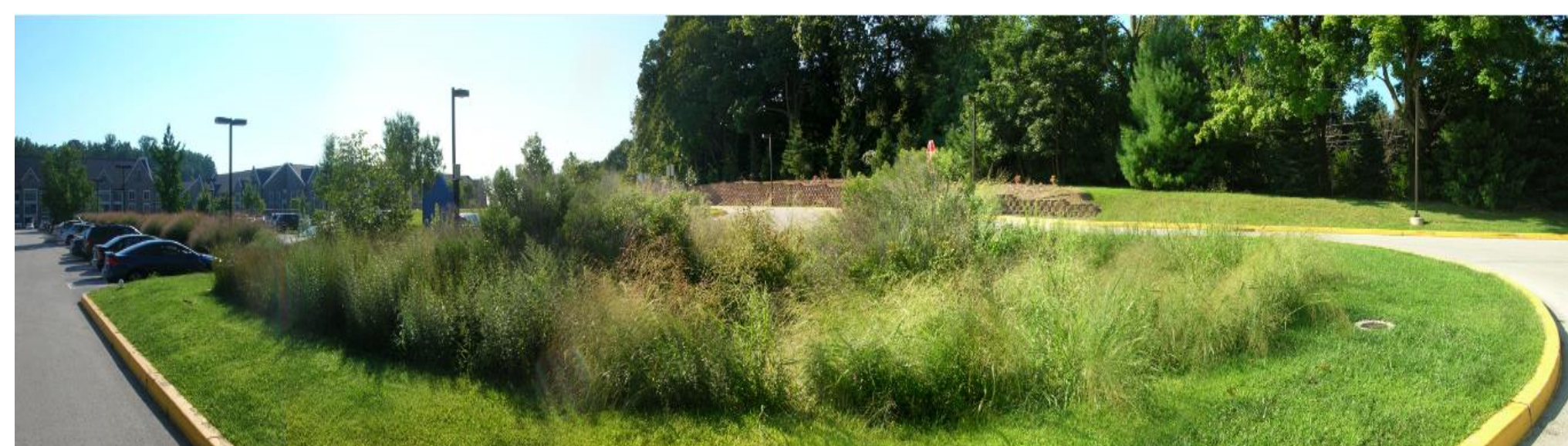
Figure 3: The Bioinfiltration Traffic Island.
